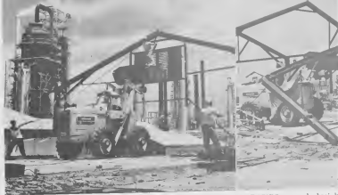
ERECTED ELEVEN years ago as a temporary fix for TSD-EIG personnel was this steel-frame structure. After relocating lab equipment and furniture, building was dismantled and moved to the barge dock where it was re-erected for Storehouse use. EIG personnel moved to new Administration Building offices.
